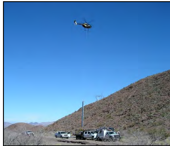
Photograph 2-6 Example of Helicopter Delivery to Structure Site
