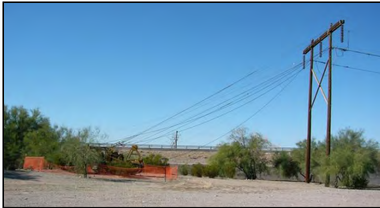
Photograph 2-9 Example of a Pulling Station
