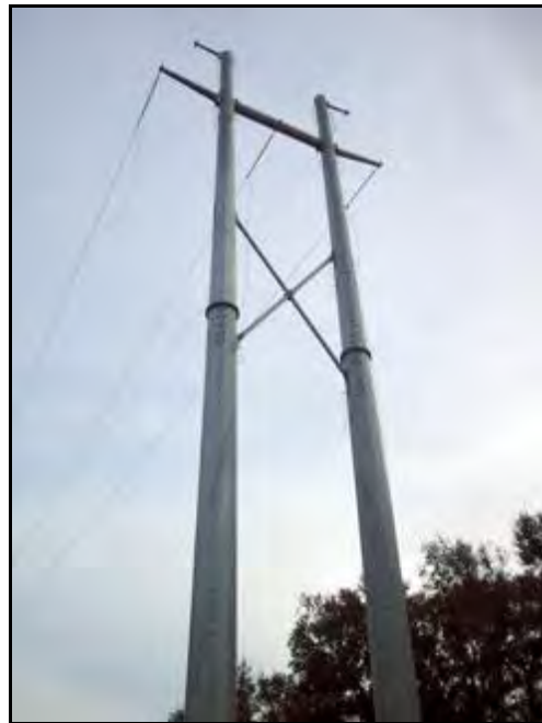
Photograph 2-3 Example of a Metal H-frame Structure (not rusty appearance)
