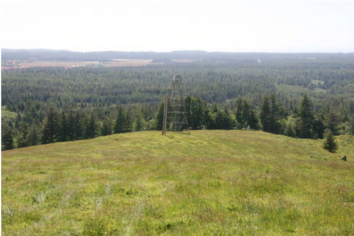
Figure 3.3-2. View of Bandon-Rogue Transmission Line from Stonecypher Road
