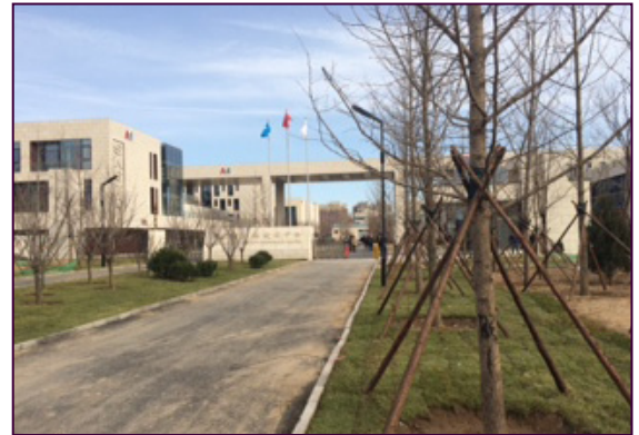
Main entrance to newly opened facility.
