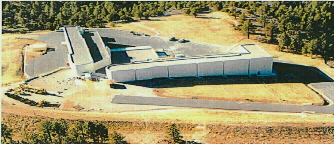
An aerial photograph of the Los Alamos DARHT facility.
