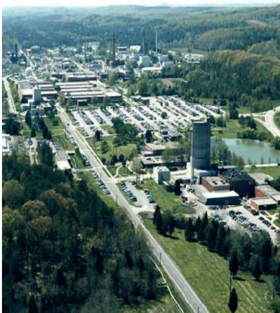
Aerial View of ORNL
