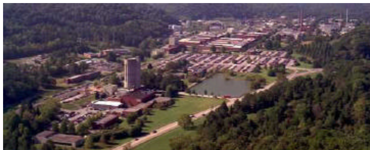
Aerial View of ORNL
