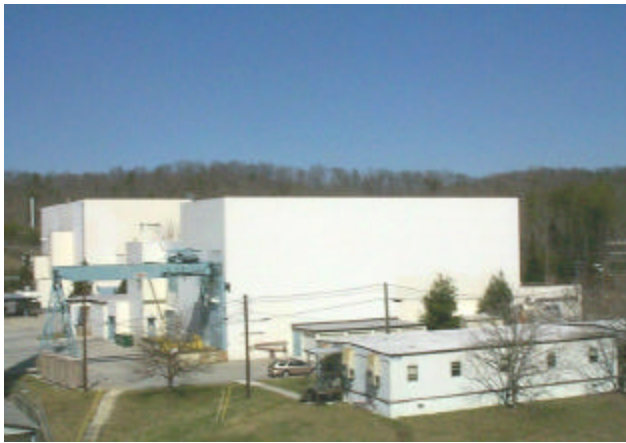
Building 7920 at ORNL
