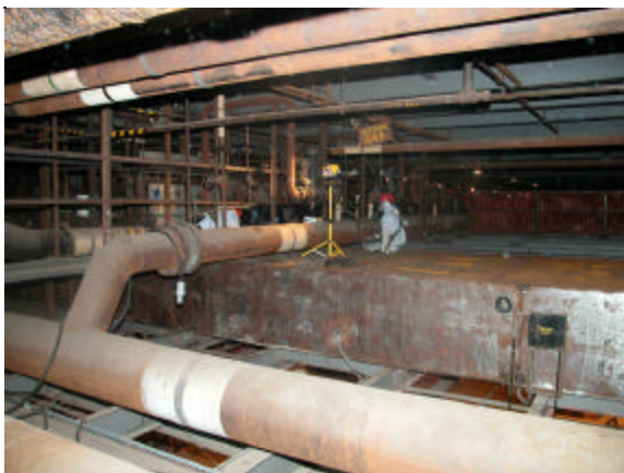
Hazardous Material Abatement in K-25
