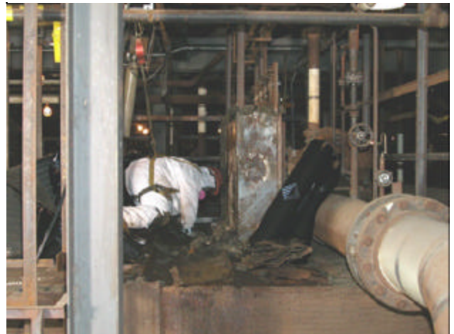
Removal of Material in Pipe Housing Area
