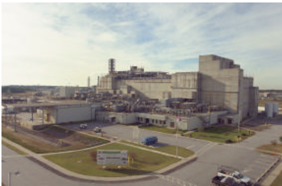
Defense Waste Processing Facility
