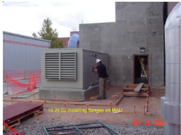
Modifications to the Bunker at MDL
