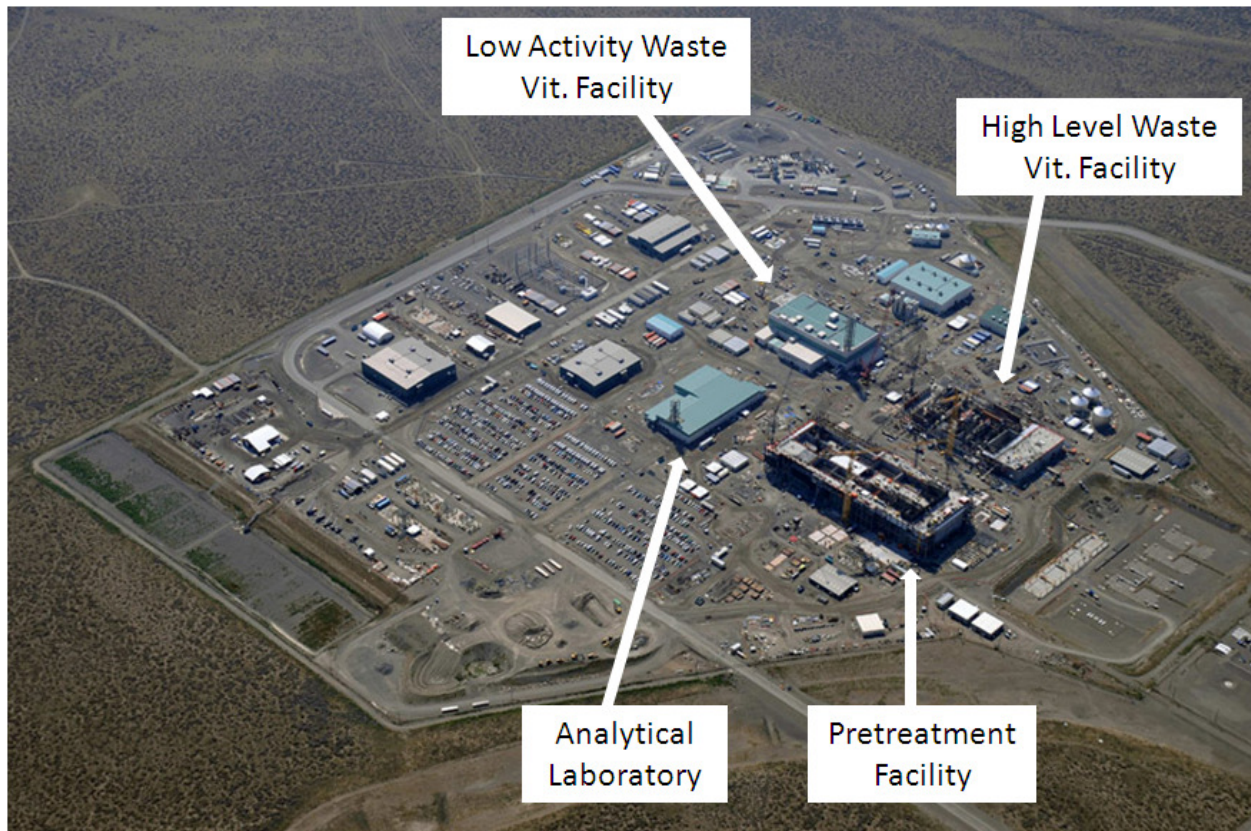
Aerial View of the WTP Construction Site, July 2010
