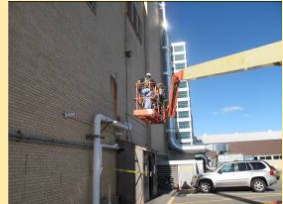
Removal of Building 701 Fan FN-002 Electrical Conduit - Nov. 3, 2009
