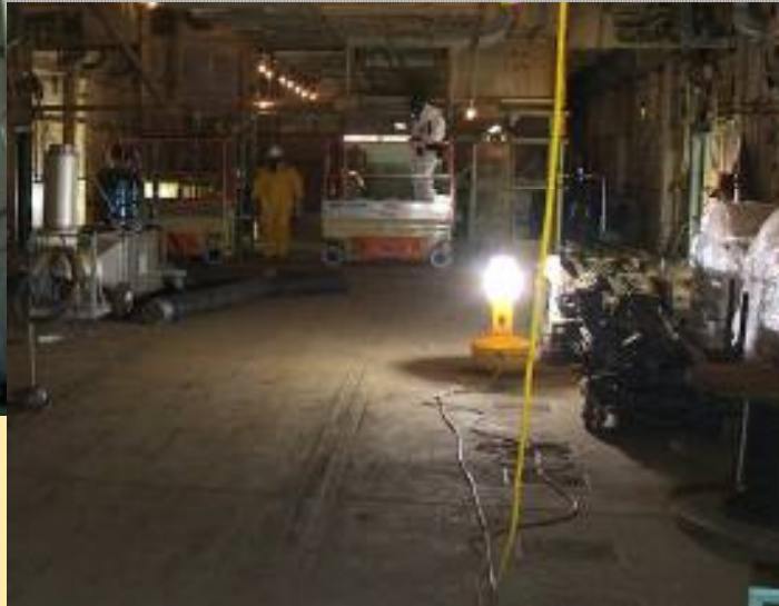
C-410 Feed Plant
