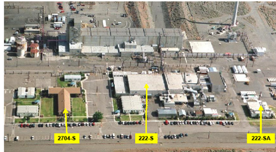
Buildings identified above are used by small business and shared with Tank Operations Contractor.
