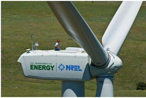
DOE 1.5MW research wind turbine installed at the National Wind Technology Center (NWTCC) in Colorado
