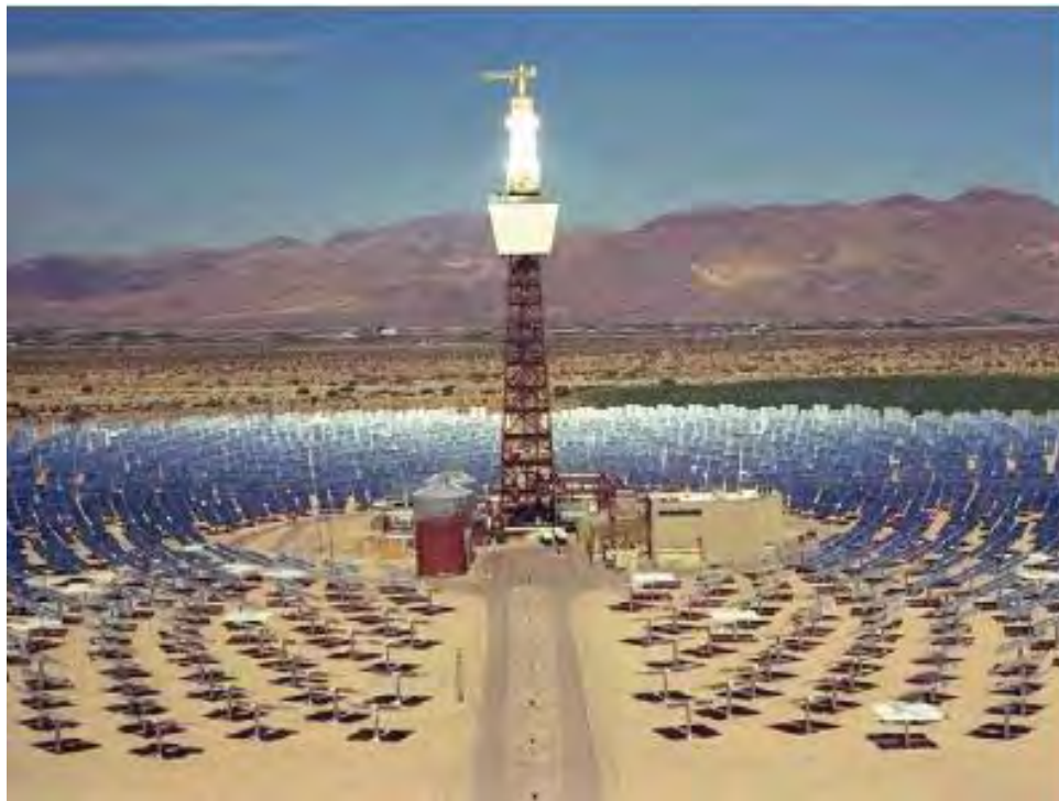
Solar Power Tower (from ISEGS PSA, 2008)
