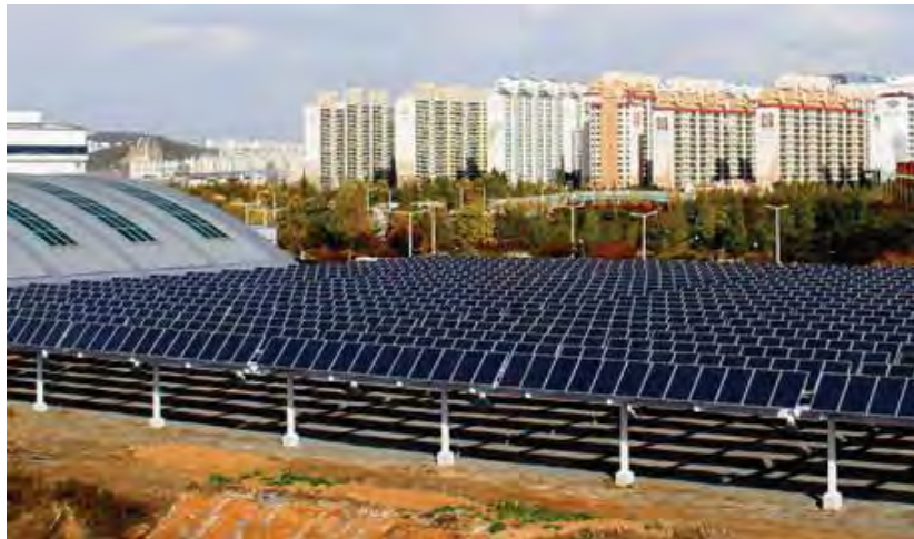
SunPower's PowerTracker Solar in Gwangju City Power Plant, South Korea - 1 MW http://www.sunpowercorp.com/For-Power-Plants.aspx
