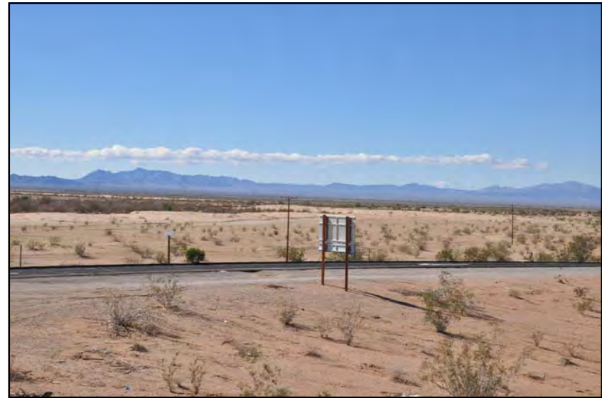
Devers-Palo Verde Transmission Line, Looking Southwest from Wiley's Well Road
