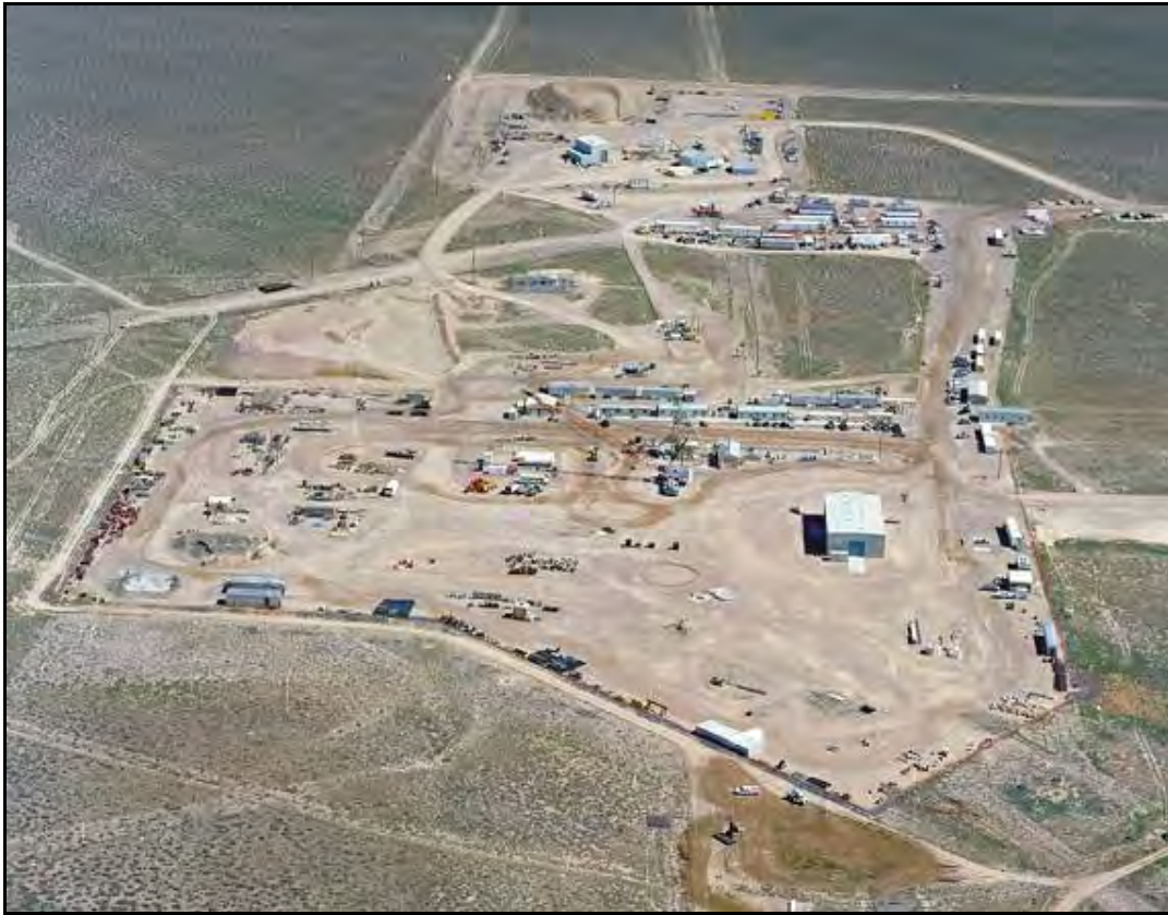
Figure 2-3 Aboveground Facilities of the U1a Complex
