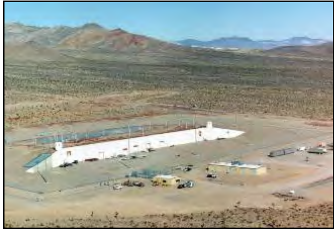
Figure 2–5 Device Assembly Facility at the Nevada National Security Site
