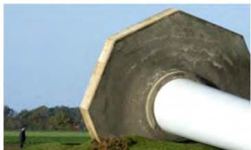
Turbine fire in France 9-19-10
