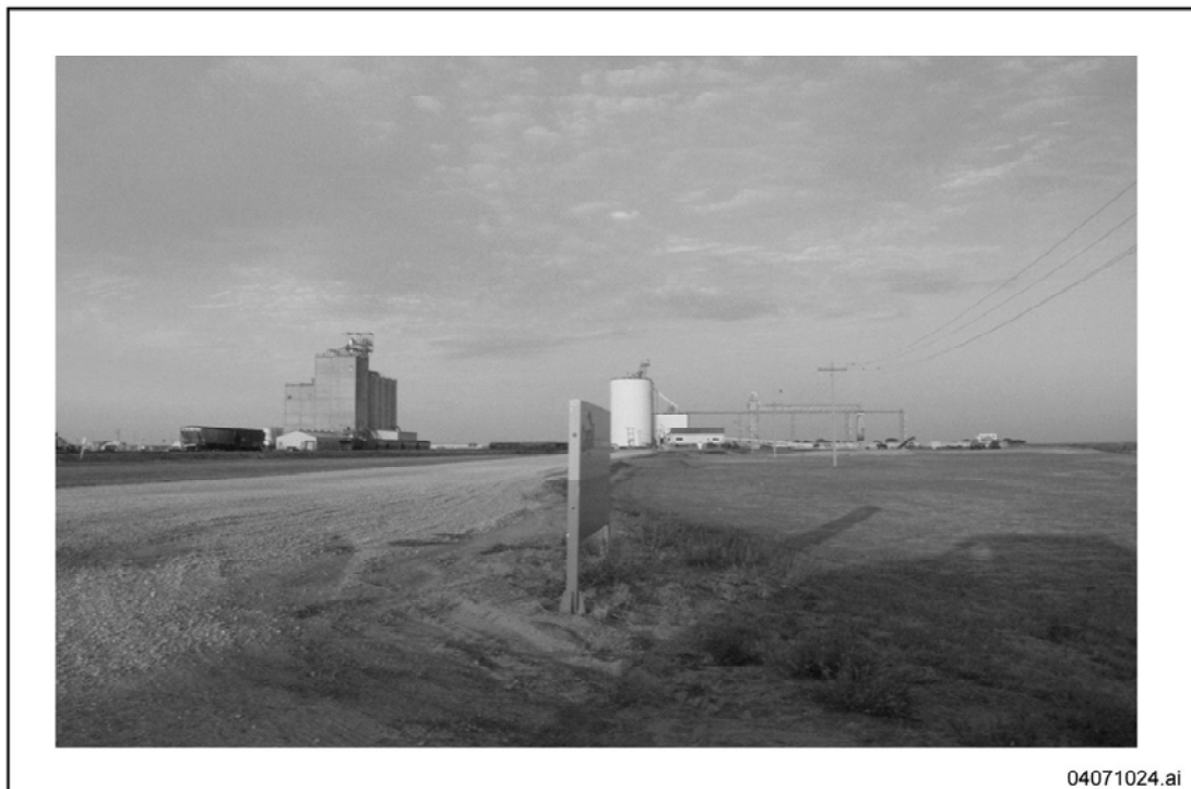
Figure 4-5. View of structures at Cargill and Seaboard Farms.
