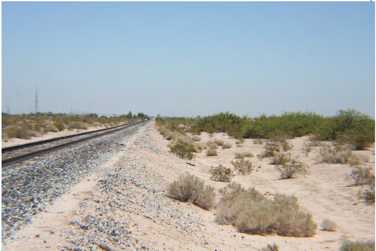
Union Pacific Railroad on Northern Boundary of North Project Parcel
