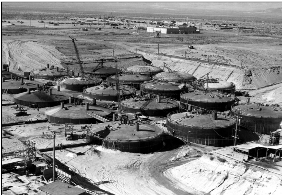
Figure S–2. Single-Shell Tanks Under Construction at the Hanford Site, 1947 to 1948
