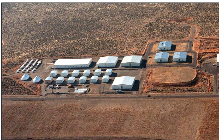
Figure S-8. Aerial View of the Central Waste Complex
