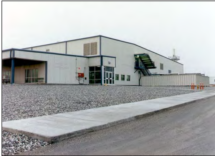
Figure S-10. Waste Receiving and Processing Facility
