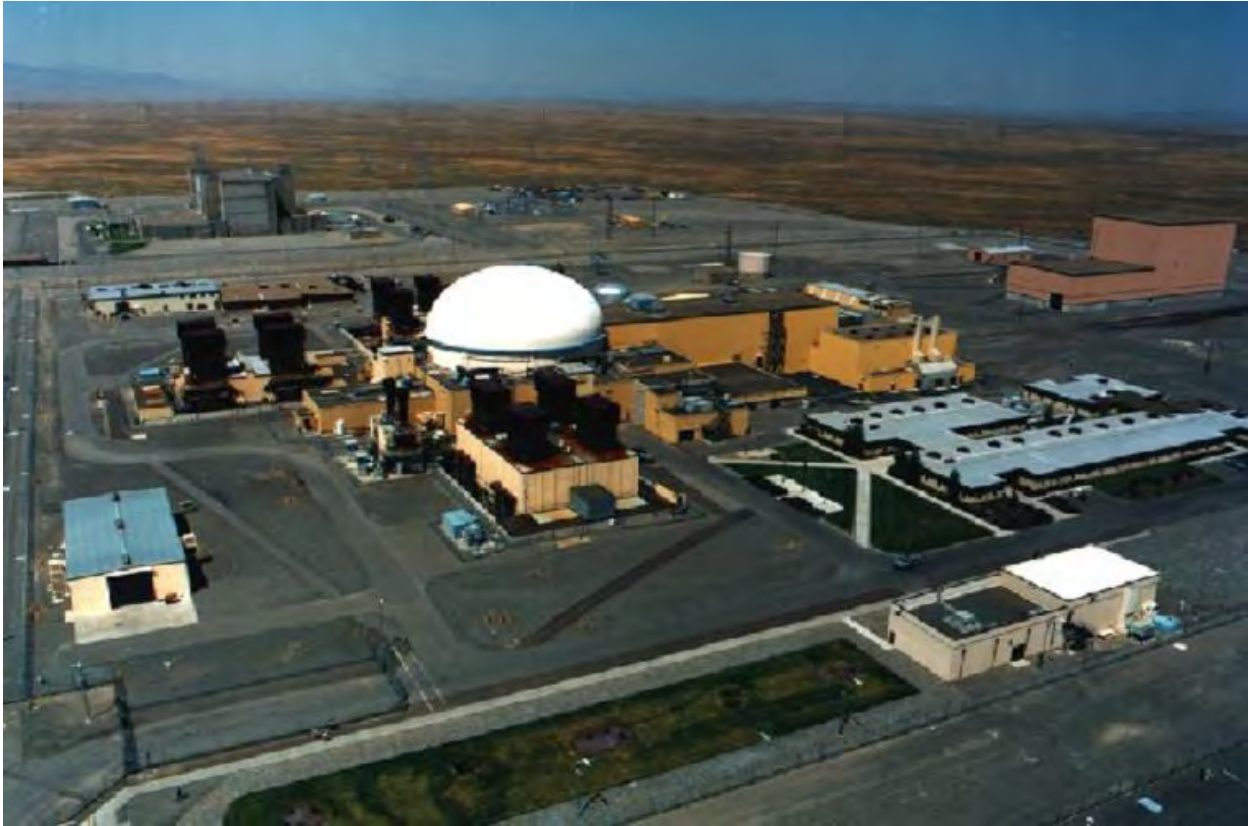
Figure S–6. Fast Flux Test Facility Complex
