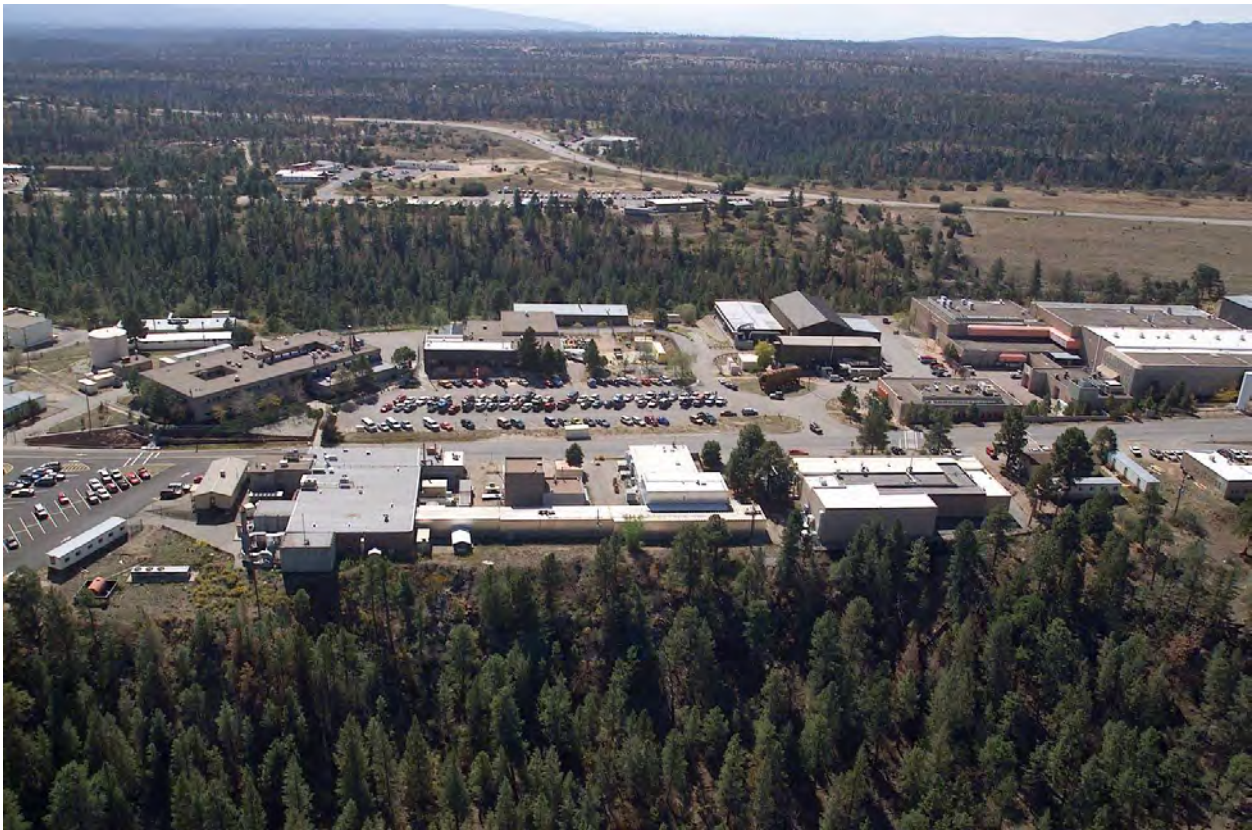
Figure J–5 Photograph of Canyon to be Bridged between Technical Area 35 and Technical Area 63
