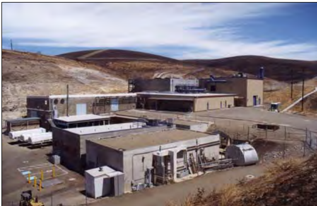
Figure A.9-2—The Contained Firing Facility at the Building 801 Complex
