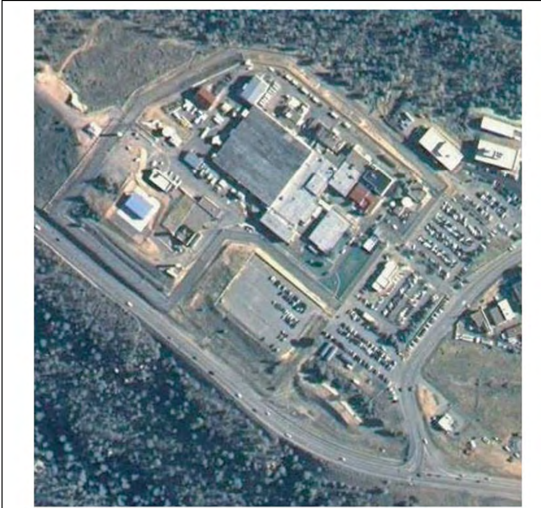
Figure A.5.1-5—Plutonium Facility at TA-55
