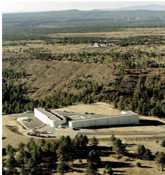
Figure 3.11-4—The DARHT at LANL
