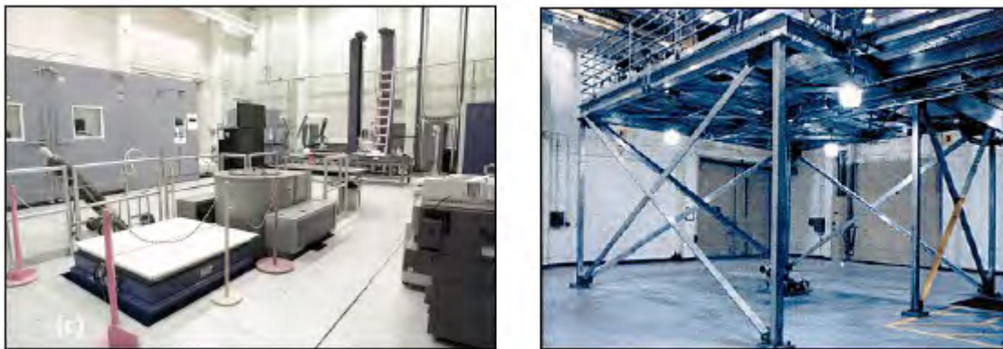
Figure 3.12-1—Photos of Building 334, Hardened Engineering Test Building (left to right): view of environmental test facilities bay and view of INRAD bay
