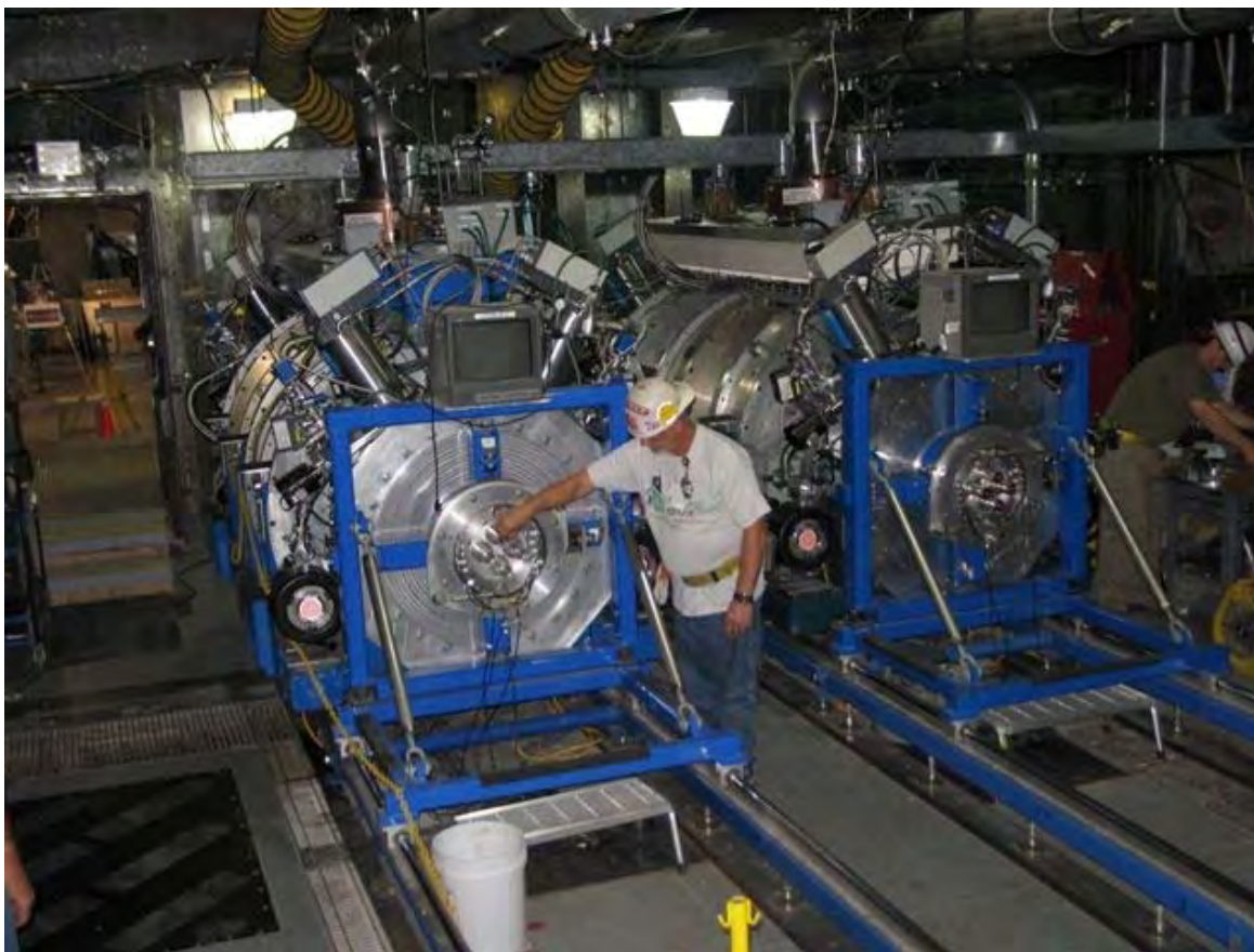
Figure 3.12-3—U1a Complex Environmental Test Facility at NTS
