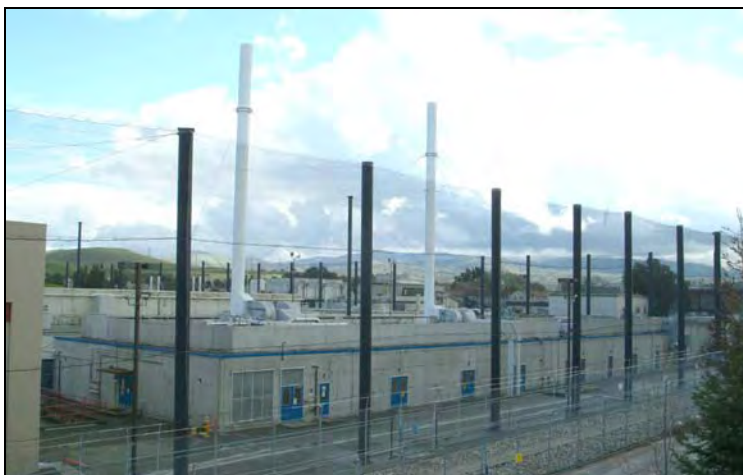
Figure 3.9-1—LLNL Tritium Facility
