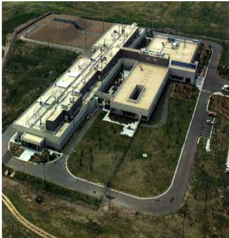
Figure 3.8-3—Explosive Component Facility (ECF); SNL/NM Bldg 905
