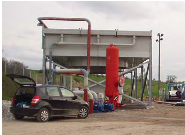
Figure 10: Cooling Fans Used in EGS Circulation Testing at Soultz, France. Shown Here Prior to Installation, These Would Be Positioned Over or Adjacent to the Heat Exchangers for Operation.
