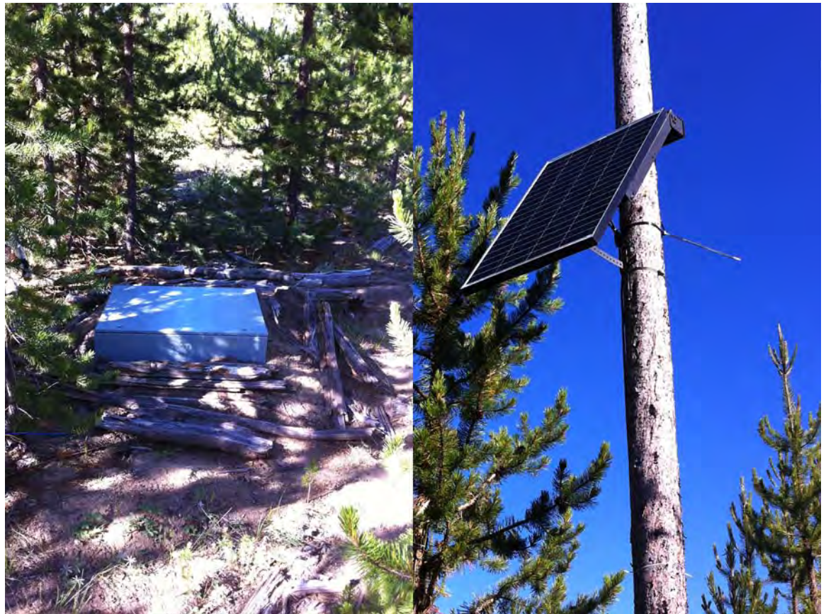
Figure 4: Typical MSA Station with Solar Panel And Telemetry Antenna
