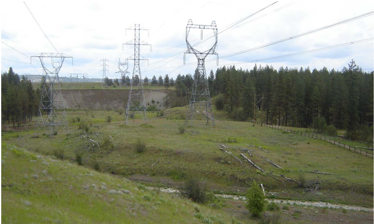
Figure 3-7. Looking East from West Seven Mile Road at Riverside State Park
