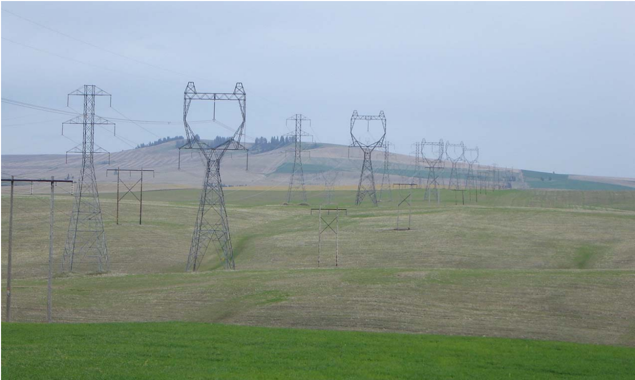
Figure 3-5. Looking East from Zwainz Road
