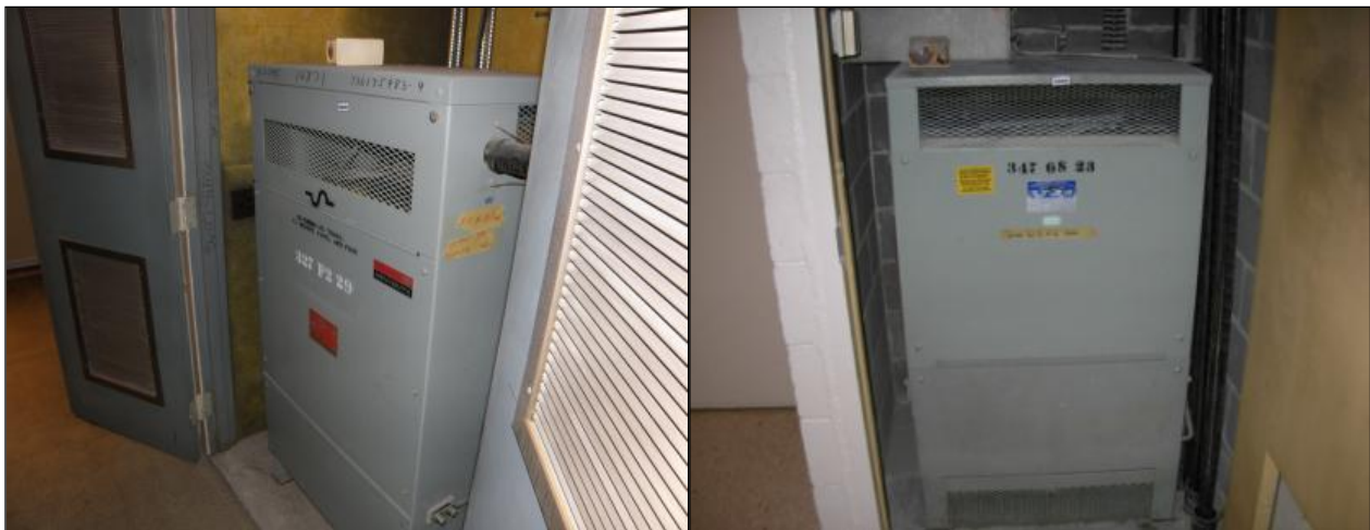
Dry type transformer installation
