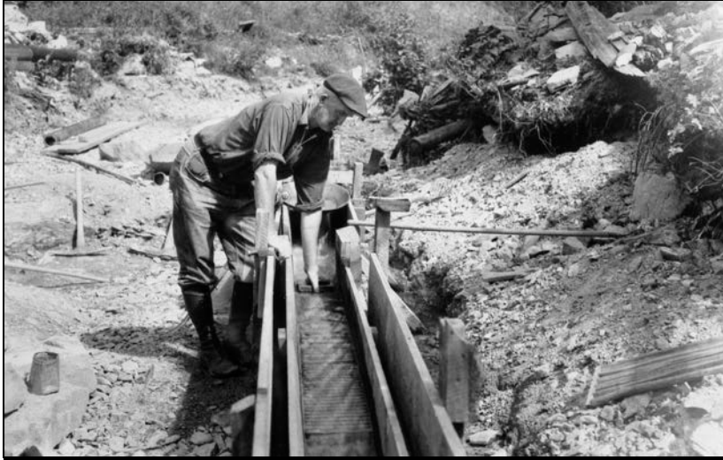
Figure 3-37. Miner at work using sluice box in north-central Idaho.
