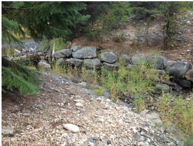
Figure B-1. Rock crib wall for “reconnecting” the river (on the left) to a pond (out of the frame on the right).
