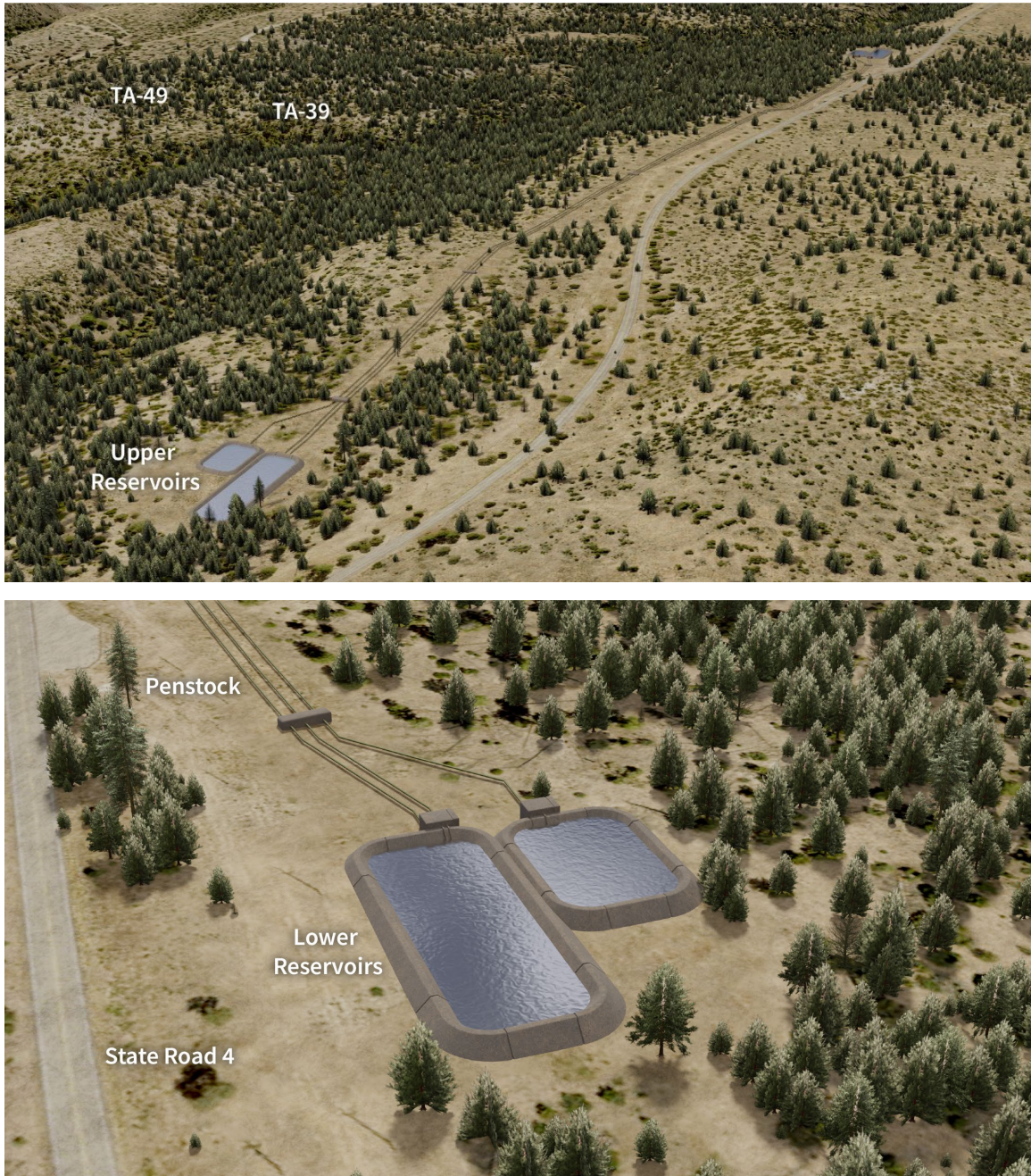
Figure 3.4-2 Pumped Hydropower Upper and Lower Reservoirs
