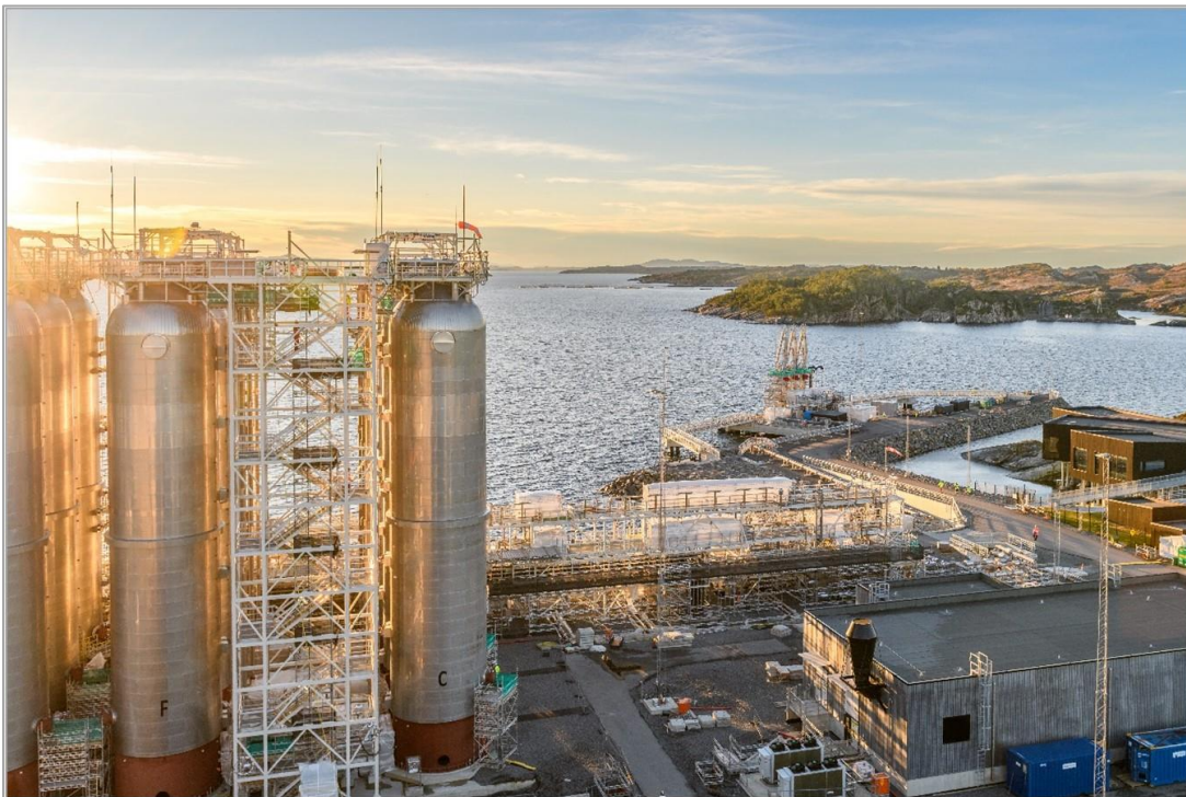
Figure 4-2. Northern Lights facilities
