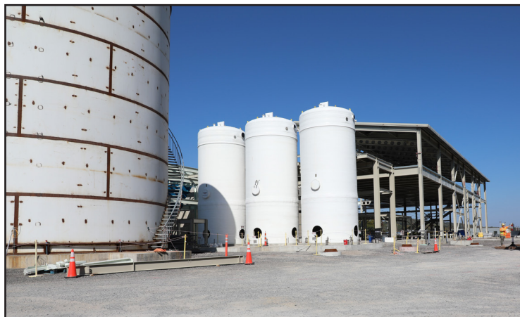
Construction progressing on the treatment plant
