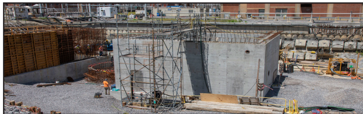
Construction progressing on the headworks facility
