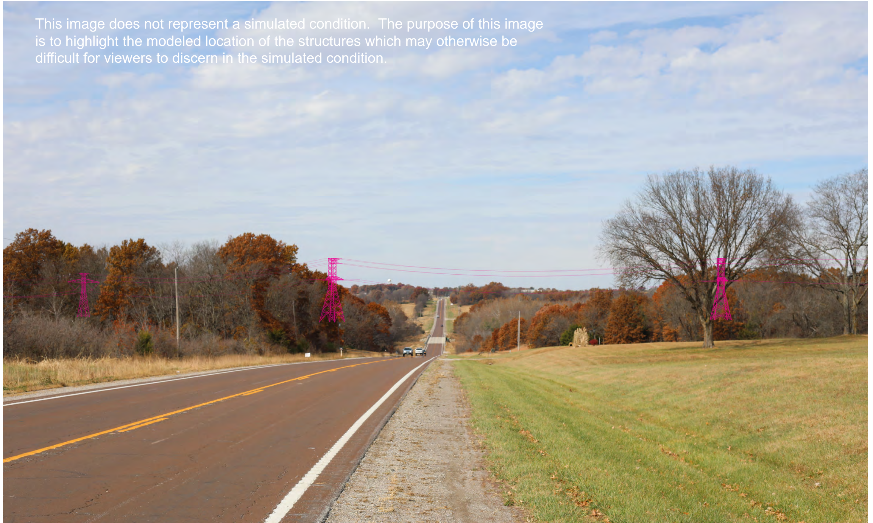
KOP 24: U.S. Highway 169 looking northwest - Color Overlay
