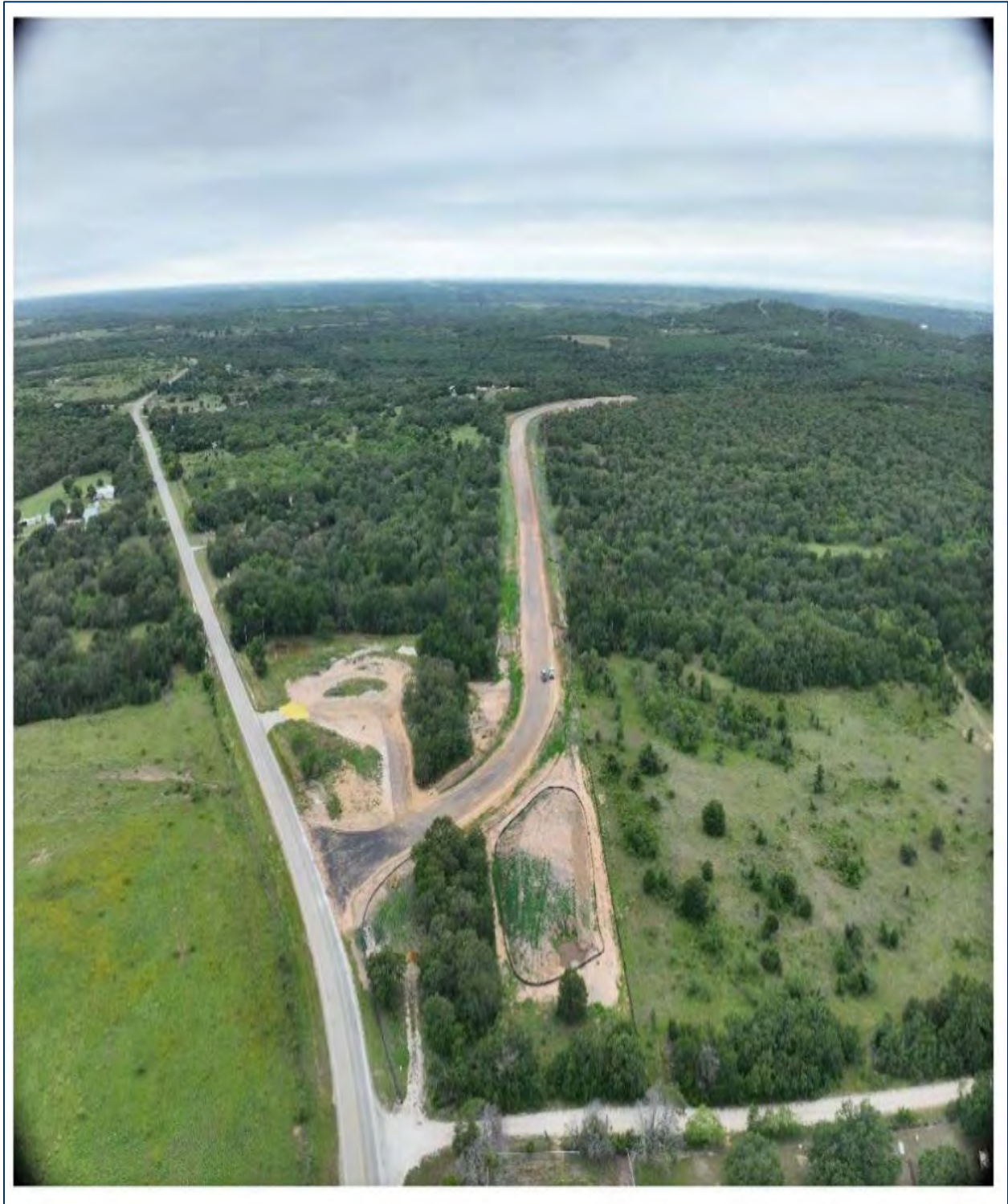
Figure 3b: Existing Conditions, May 2024, Facility Entrance/Access Road Cleared and Graded
