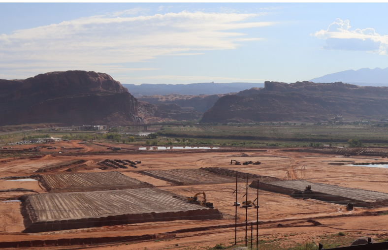
An overlook view of the Moab Site tailings pile, with rectangular drying beds.
