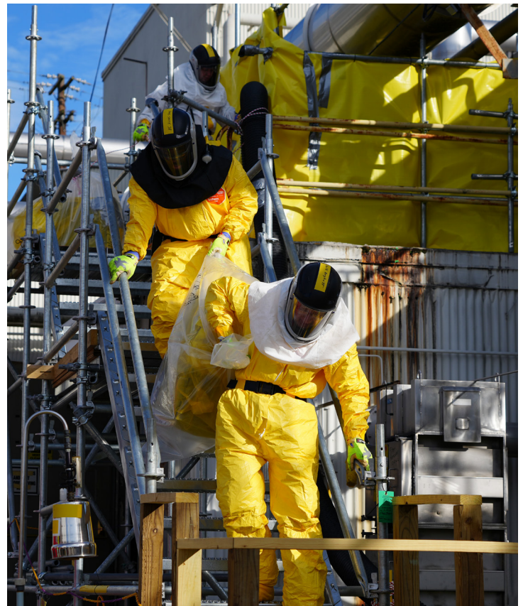
Crews perform deactivation activities at 13 ORNL buildings.
