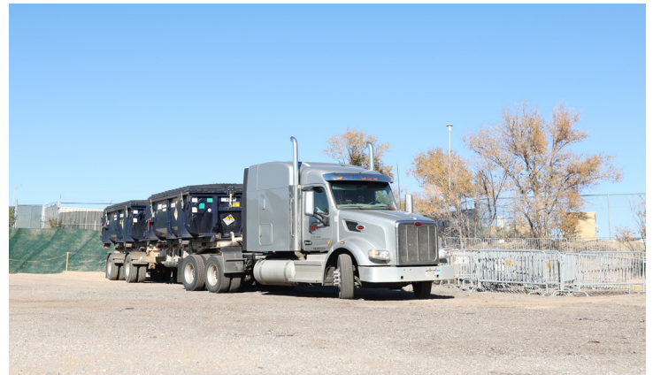
Truck carrying the final shipment of contaminated soil and debris from legacy operations leaves the Middle DP Road Site.
