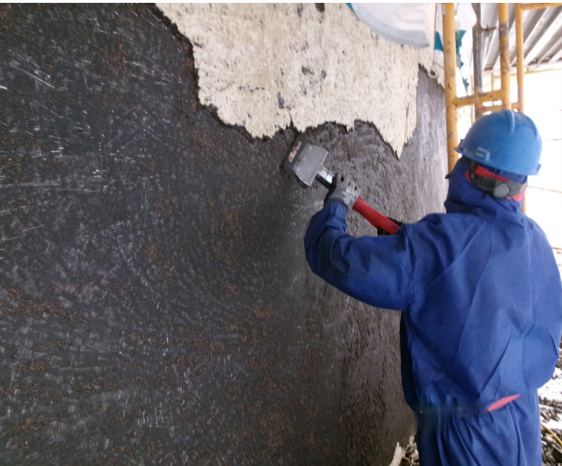
Crews remove mastic undercoating at Lawrence Livermore National Laboratory Building 280.
