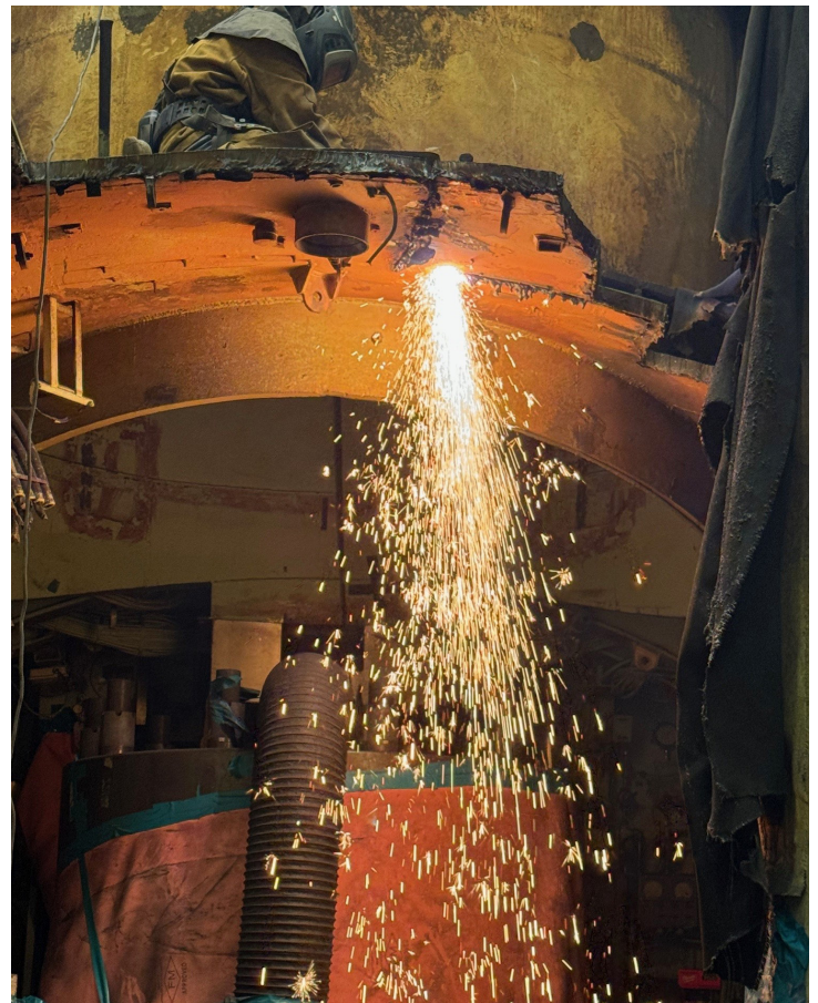
A worker uses a plasma torch to cut through a hull at the S1W prototype.
