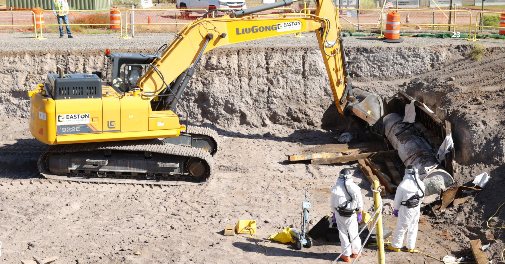
Waste Operations workers retrieve the final corrugated metal pipe containing cemented TRU waste at TA-54, Area G.
