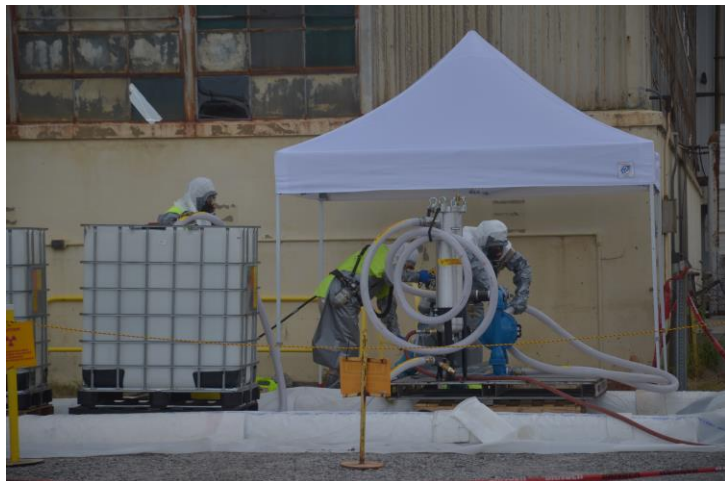
Figure 3.1. Removal of Acid Neutralization Tank Contamination
