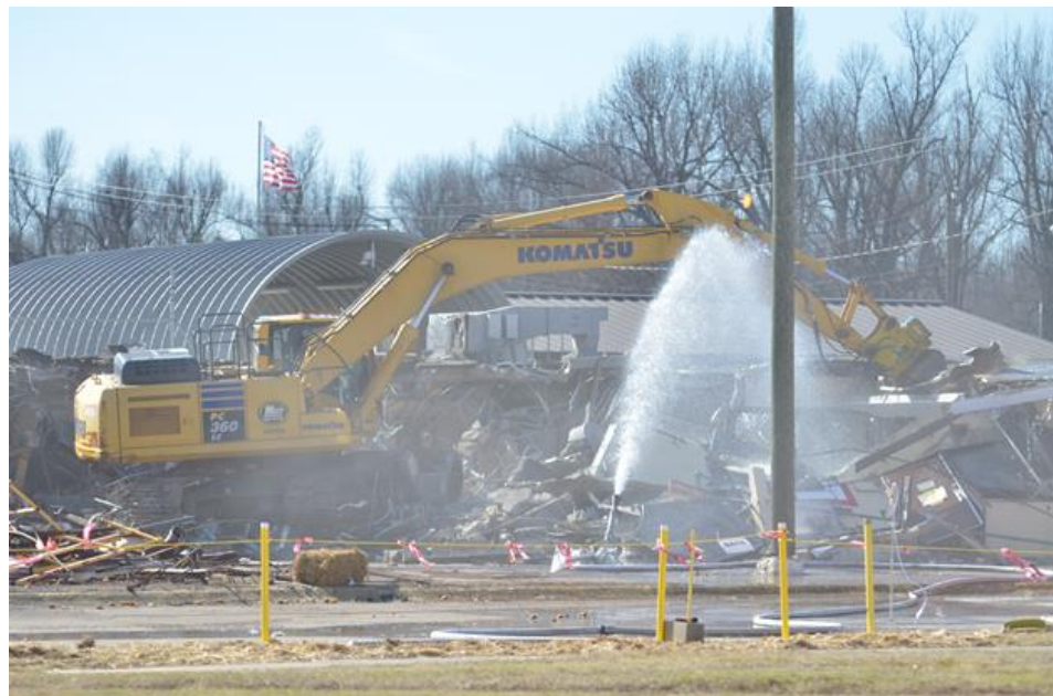
Figure 2.2. C-212 Office Building Demolition
