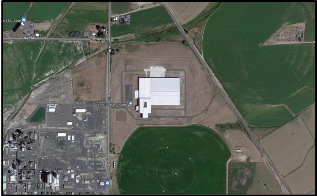
Figure 2 – Existing Site Conditions Map
