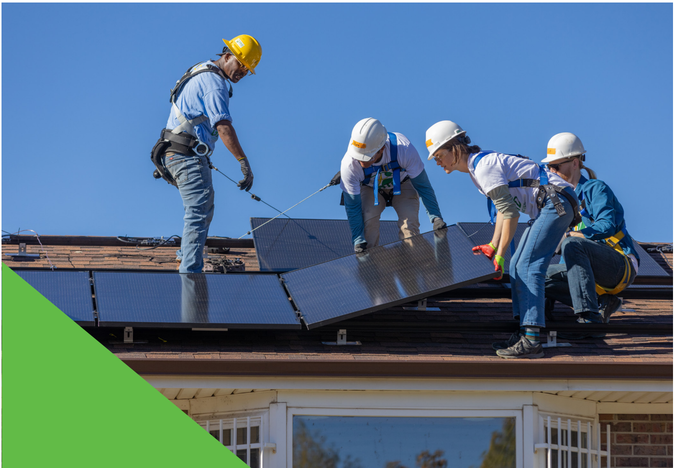
Workers install rooftop solar panels. Photo courtesy of Joe DelNero, NREL
