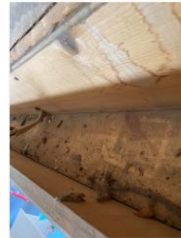
(Tribal Center) Rotunda light troughs - cleaned
