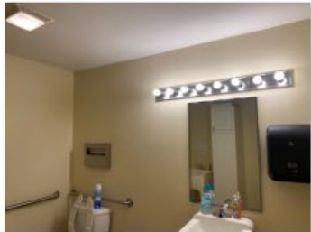
(Corporation Office) Rear bathroom vanity lights replaced
