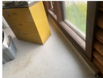
(Tribal Center) Rewired baseboard heater.
