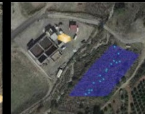
Location 2: Wastewater Treatment Plant
