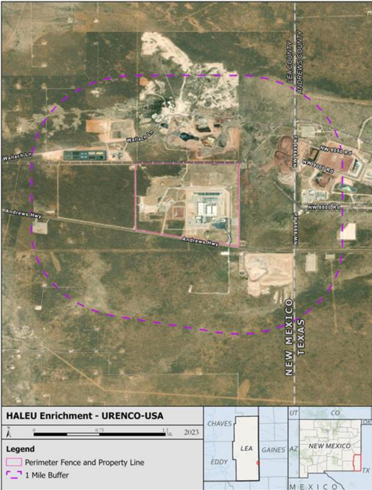
Figure 3-5. Existing UUSA Site – Eunice, New Mexico (1-Mile Buffer)
