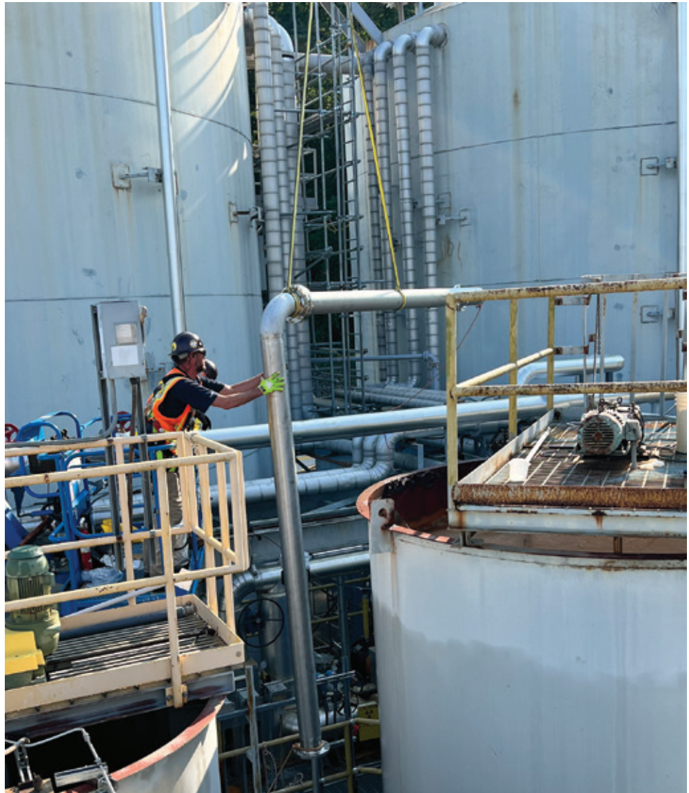
Workers install piping as part of the 3608 piping replacement project
