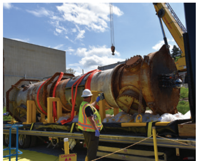
Reactor vessel loaded onto truck
