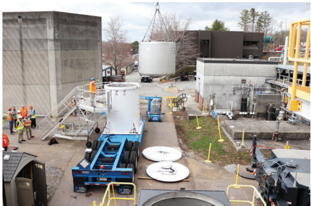
Waste tank being moved to a shipping cask
