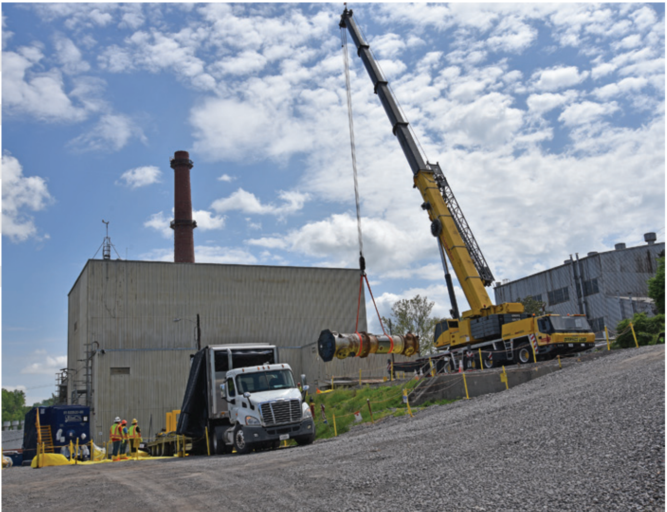
Reactor vessel being transferred to a truck for offsite disposition
