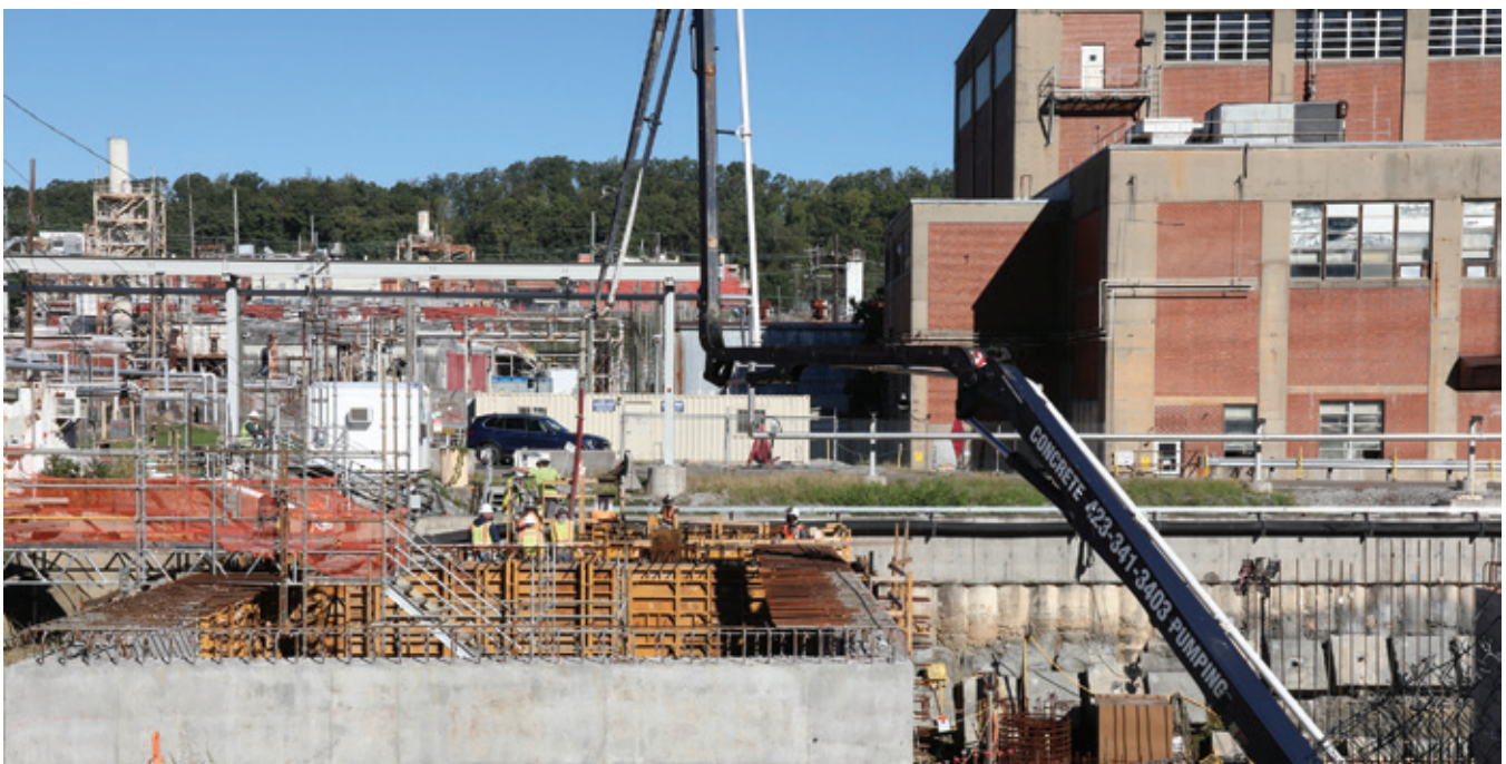
Construction activities at the Mercury Treatment Facility
