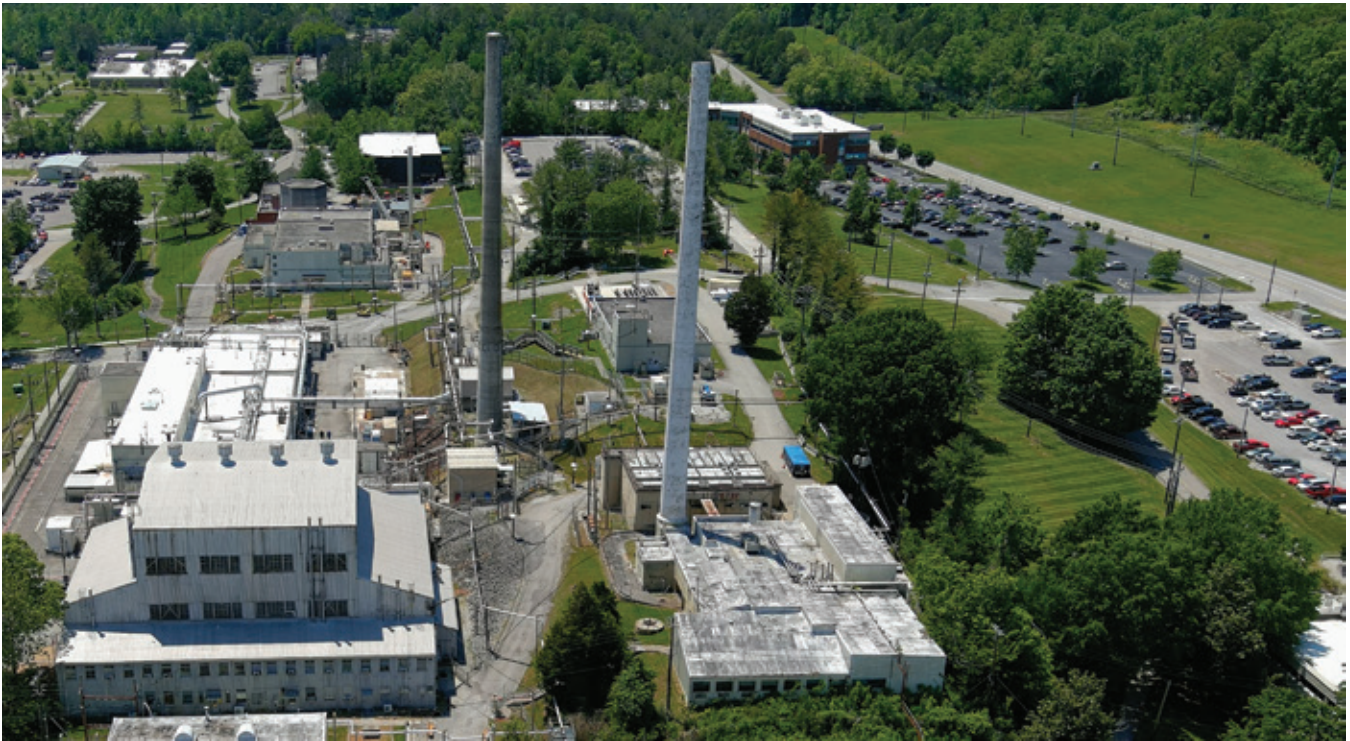
Oak Ridge Graphite Reactor and its support facilities
