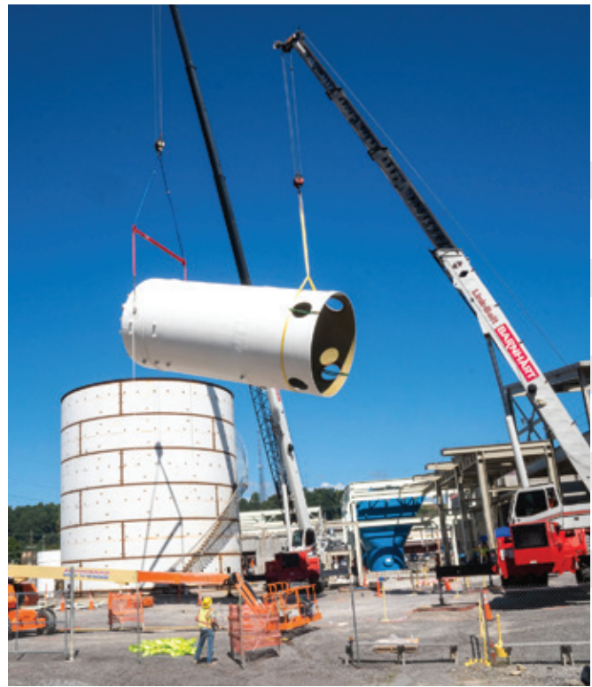
Tank installation at the Mercury Treatment Facility
