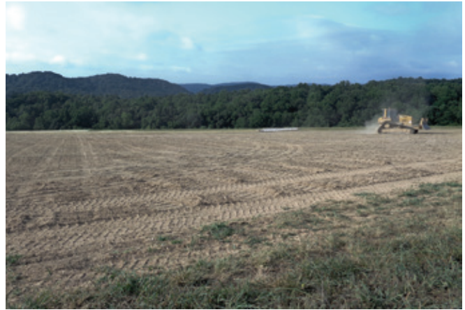
Completion of cap maintenance on Sanitary Landfill II
