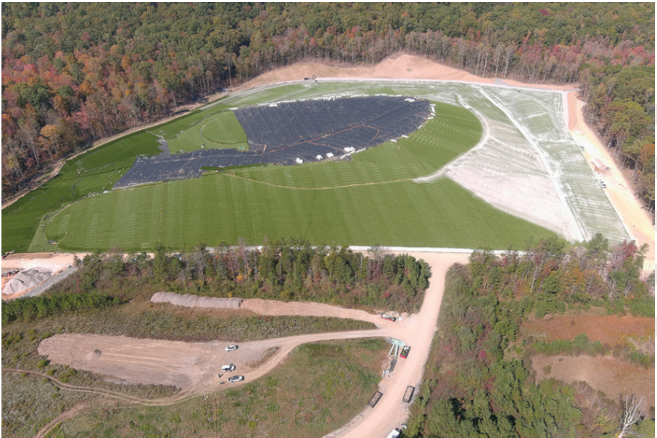
Workers made great progress on EMDF construction in FY 2024
