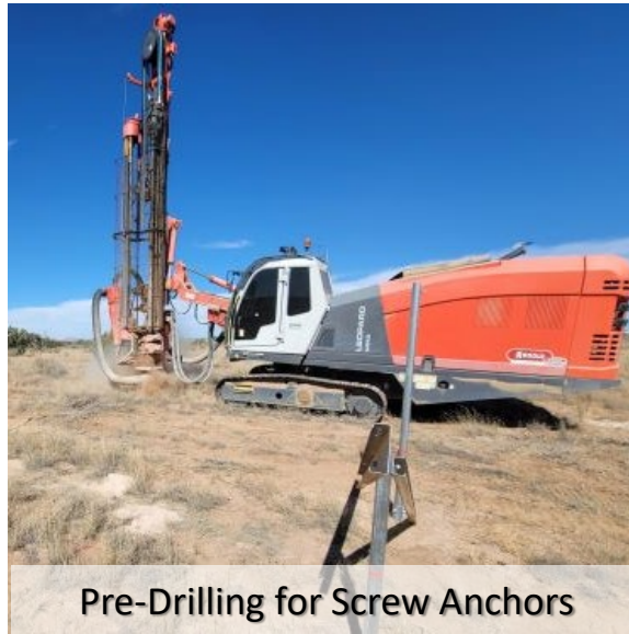
Screw Anchors for PV Module Rack
