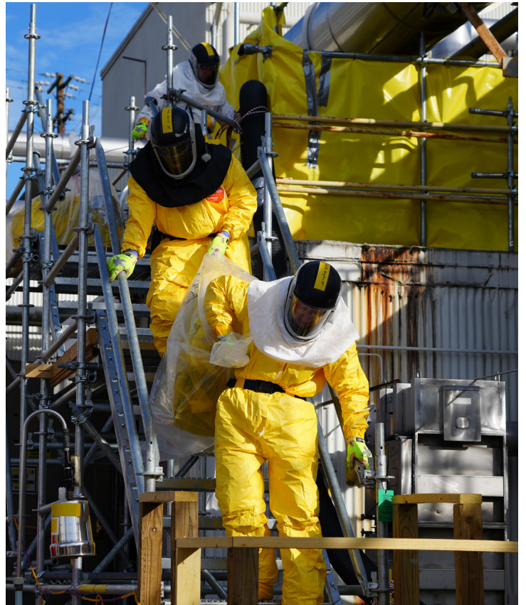
Crews perform deactivation activities at 13 ORNL buildings.
