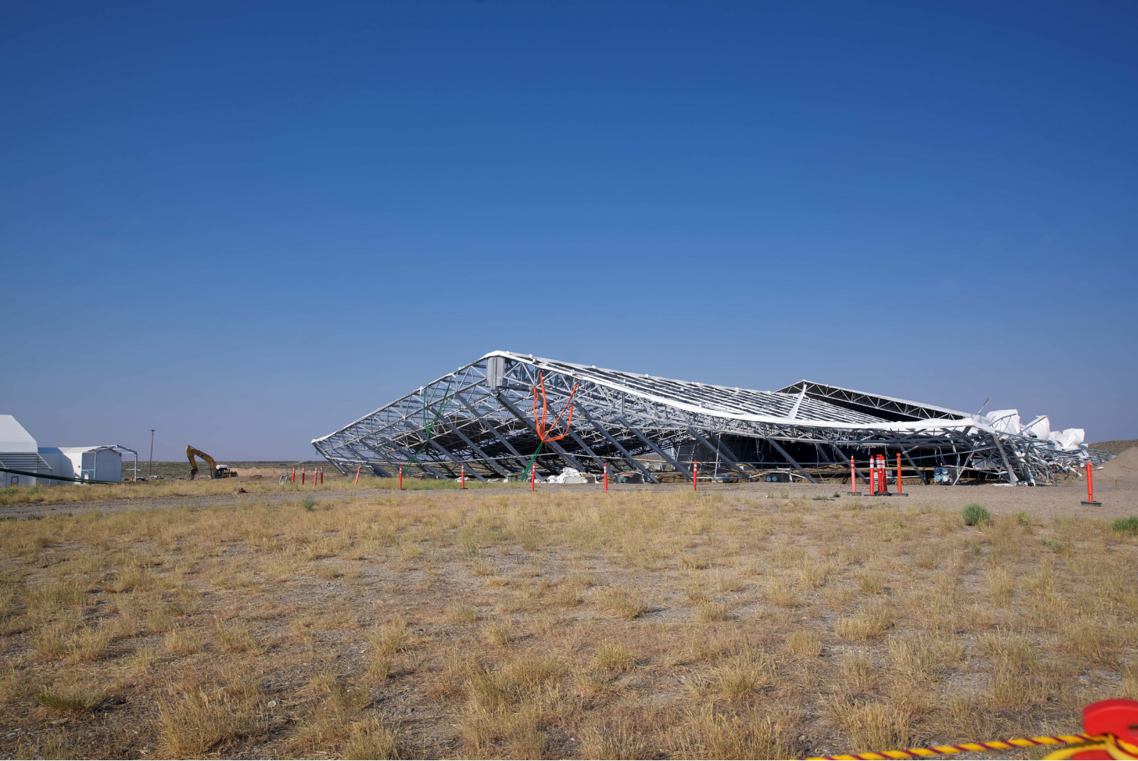
Bulldozers pull over a section of Accelerated Retrieval Project VIII.
