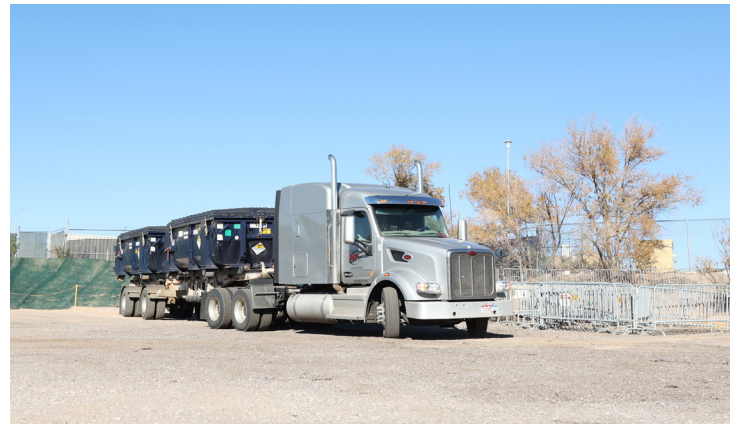
Truck carrying the final shipment of contaminated soil and debris from legacy operations leaves the Middle DP Road Site.
