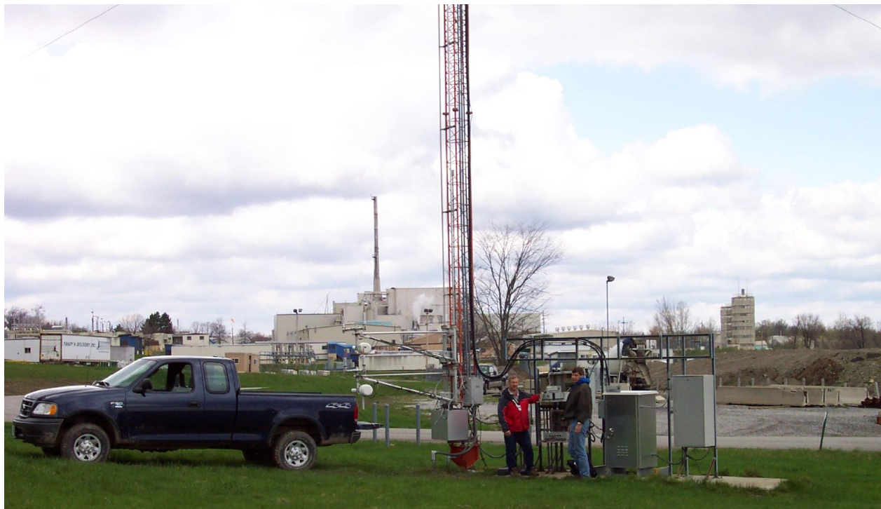
On-Site Meteorological Tower
