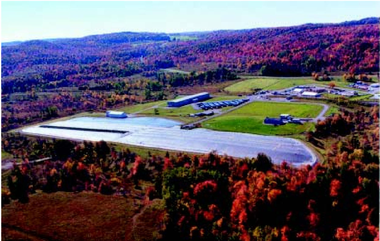
An Aerial View of the New York State-Licensed Disposal Area (SDA)
