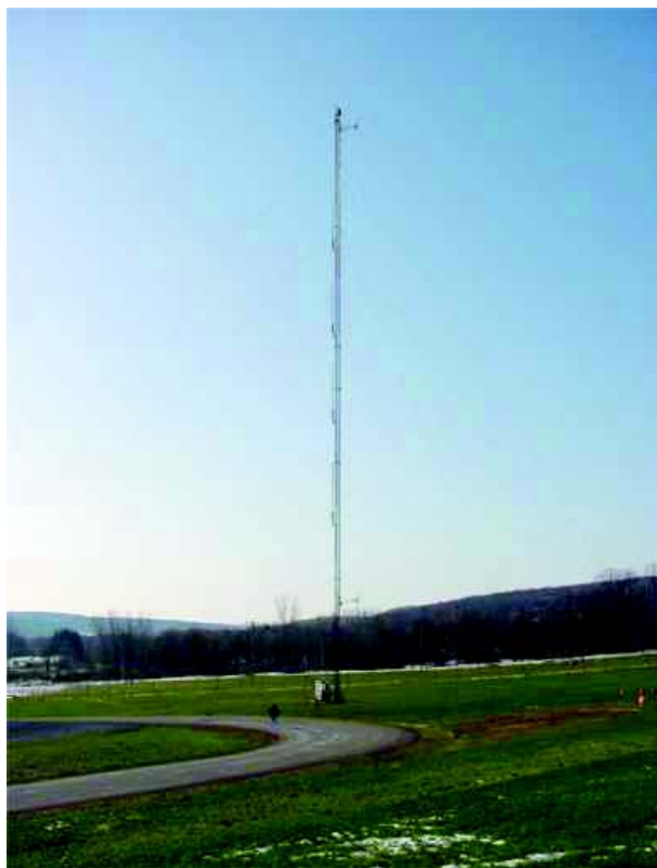
On-Site Meteorological Tower
