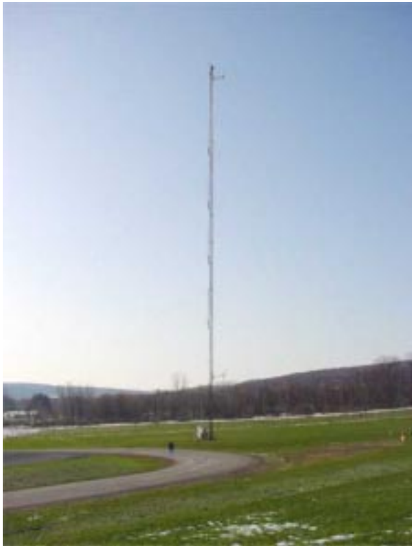
On-Site Meteorological Tower
