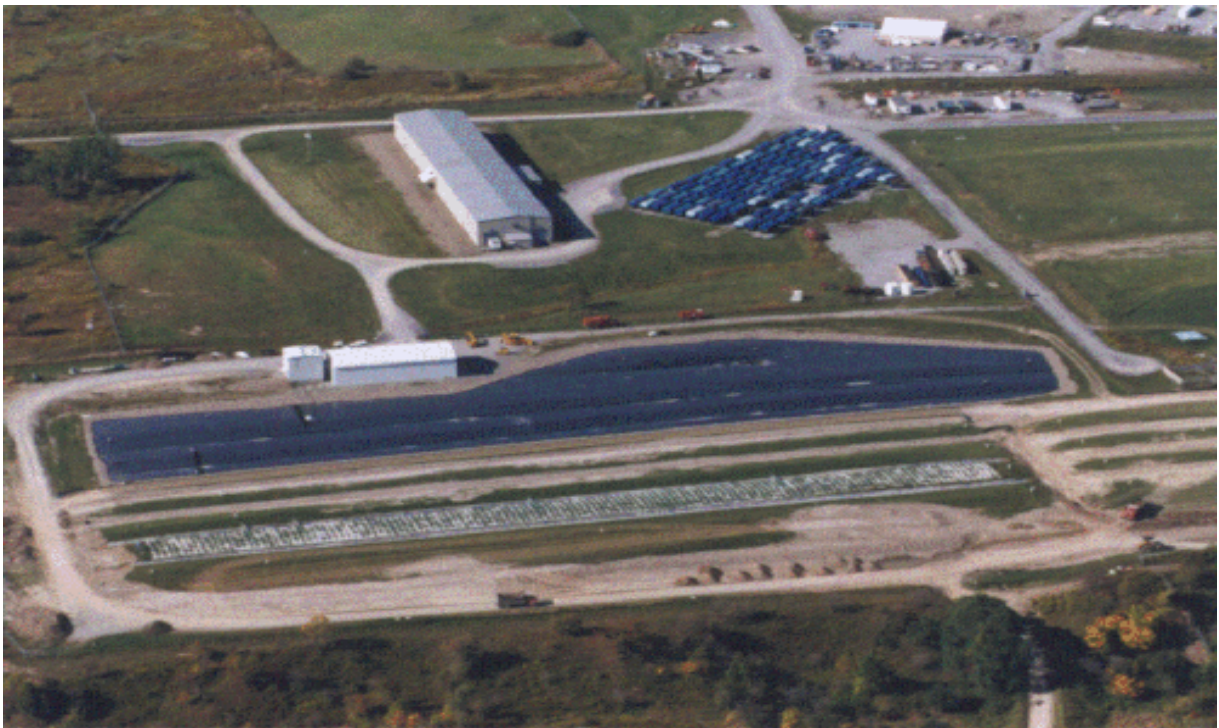
An Aerial View of the New York State-licensed Disposal Area
