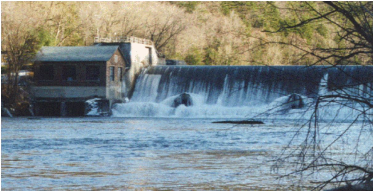
Springville Dam on Cattaraugus Creek
