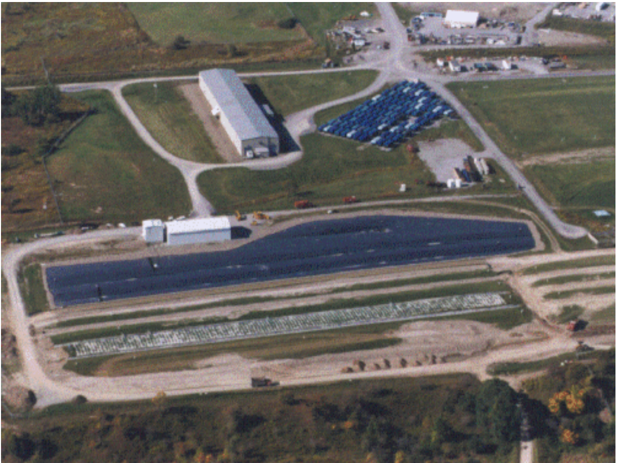
An Aerial View of the New York State-licensed Disposal Area
