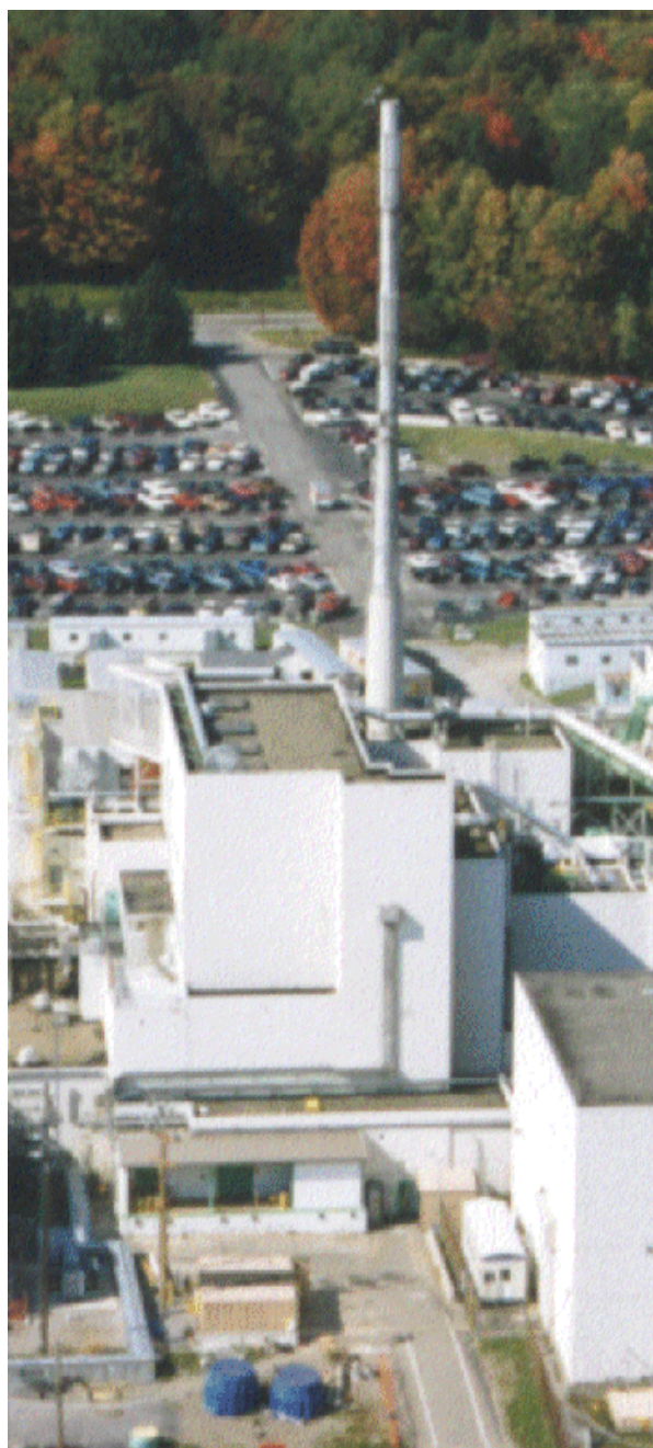
The Main Plant Ventilation Stack at the WVDP
