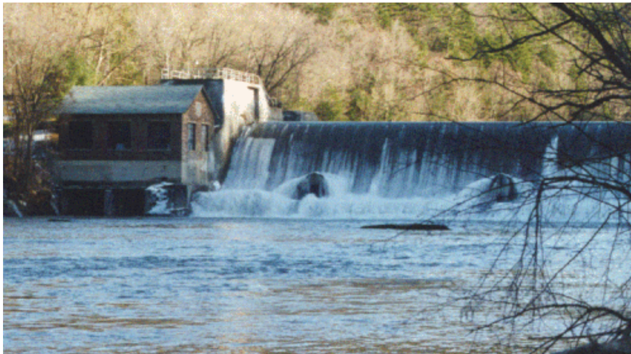
Springville Dam on Cattaraugus Creek
