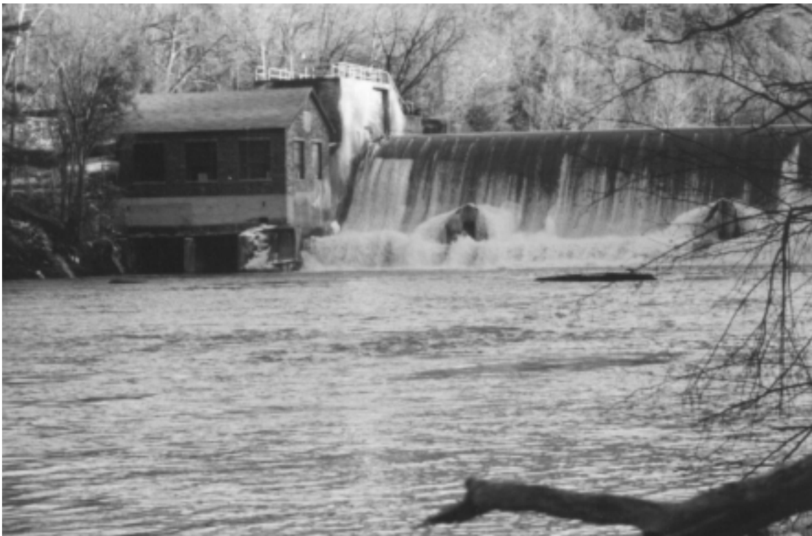
Springville Dam on Cattaraugus Creek
