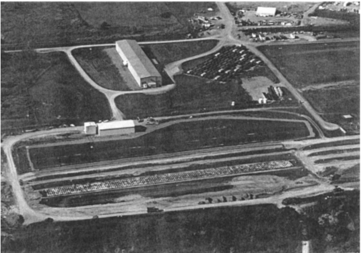
An Aerial View of the New York State-licensed Disposal Area
