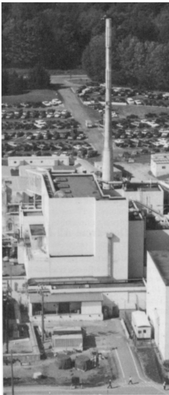
The Main Plant Ventilation Stack at the West Valley Demonstration Project
