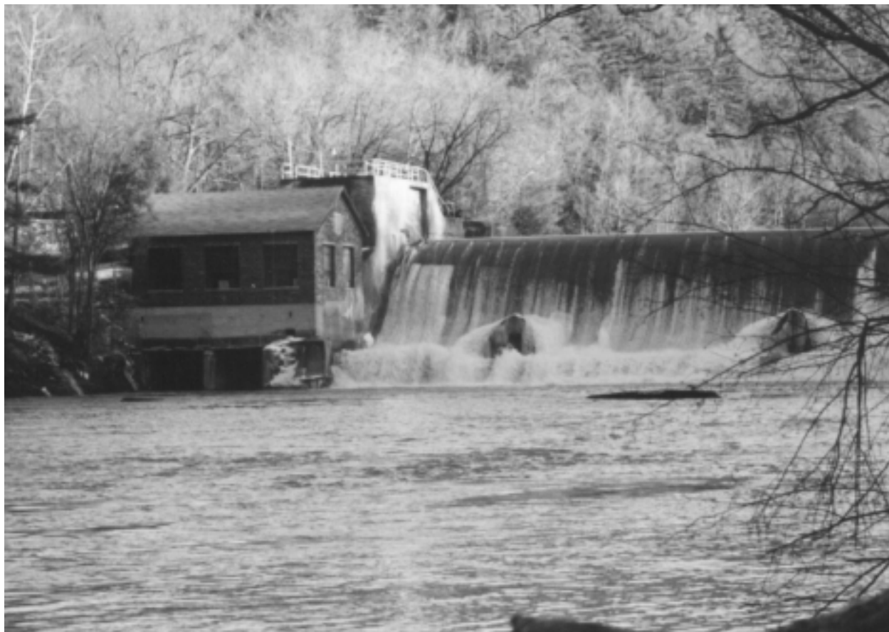
Springville Dam on Cattaraugus Creek
